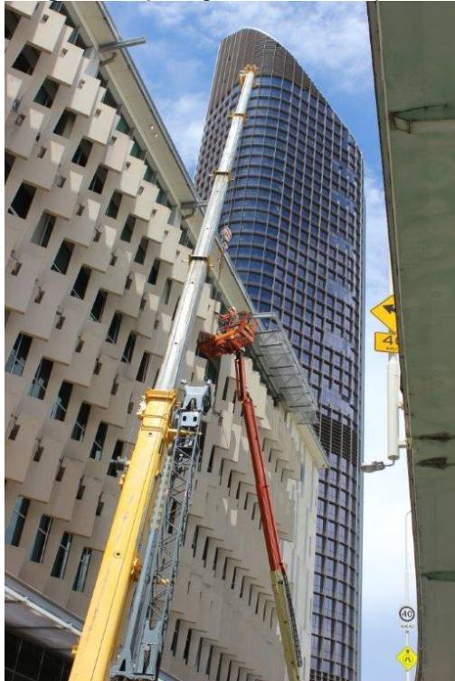
Image 1: Preparing to remove the precast concrete sunshades from the former Neville Bonner building
