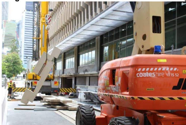
Image 2: Precast concrete sunshades lowered to the ground
